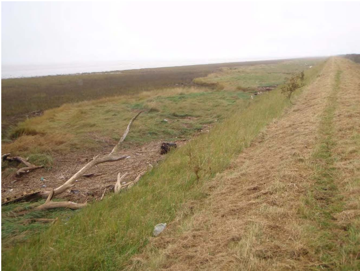
Plate 2: View of sea wall looking northwest
